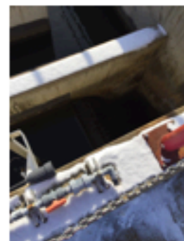
End of the line: clean water
