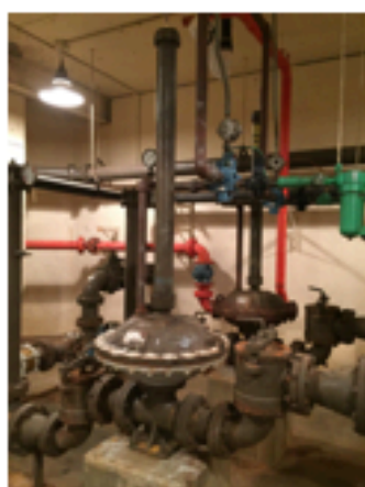
Moving the solids to the digester
